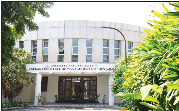
AIMS Main Building
